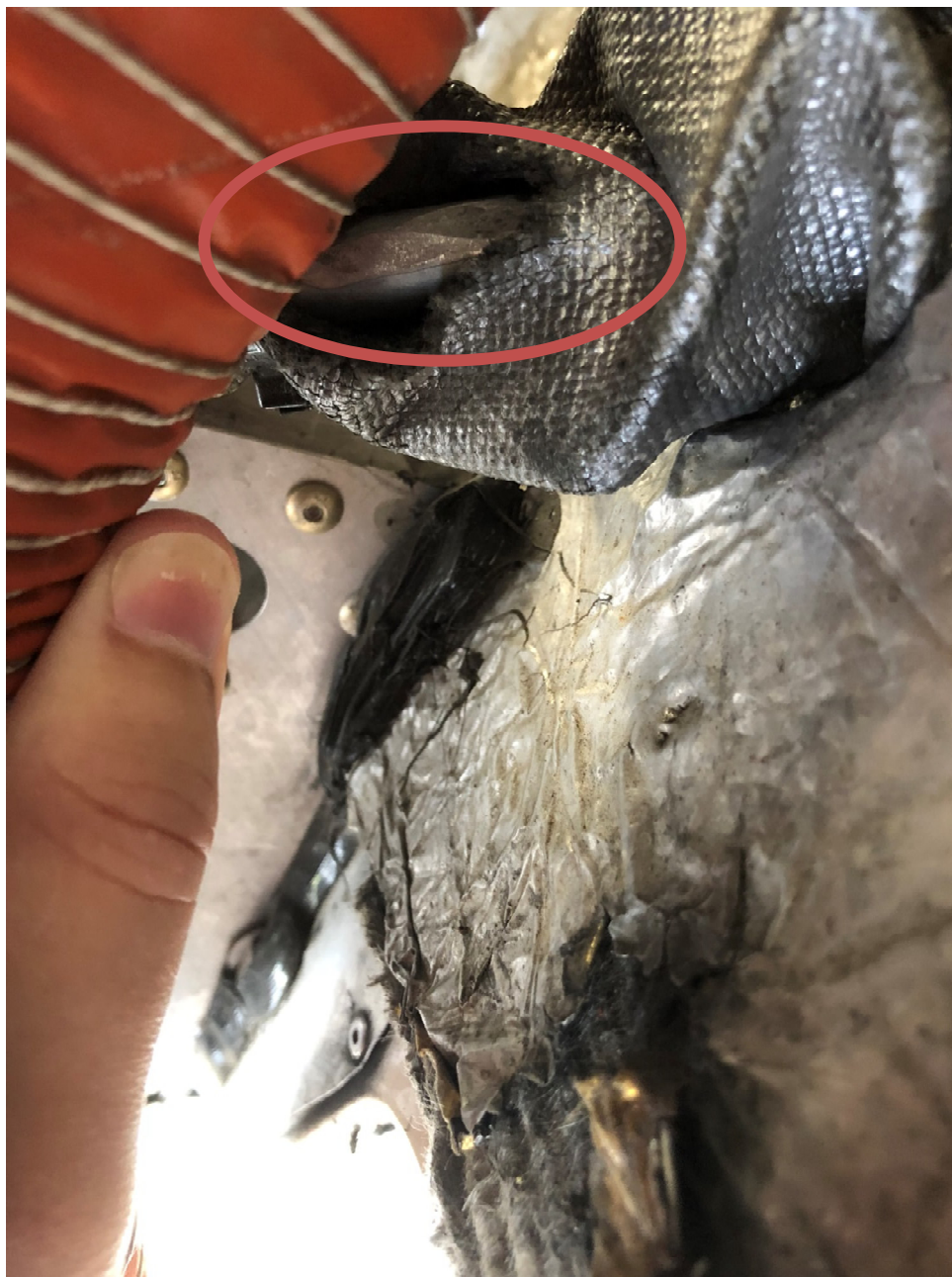
Figure 2, abrasion visible through damaged firewall boot by moving SCAT hose.
