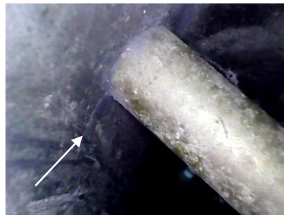
Figure 5 - photograph of crack emanating from side of hole taken with a USB endoscope
